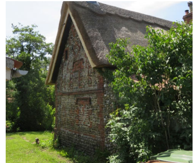
North gable end of the thatched house
