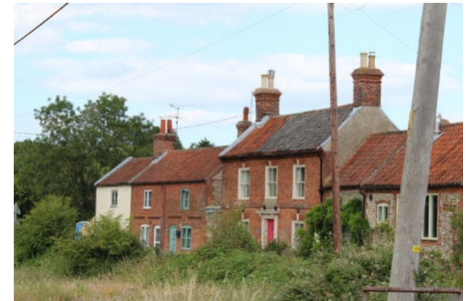
Brookside House beside Meadow Barn
