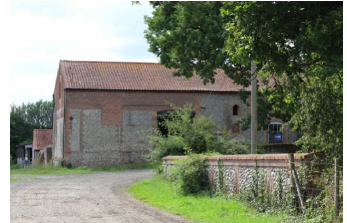
Barn range located west of Thornage Hall
