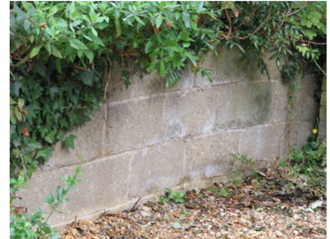
Example of a breezeblock wall
