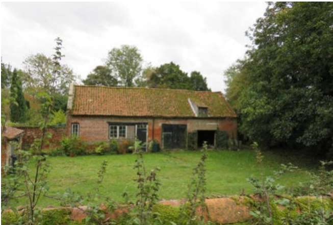
Red brick outbuilding within the land of The Old Rectory
