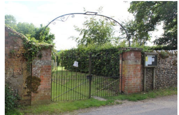
Boundary wall and entrance gate to the Church of All Saints
