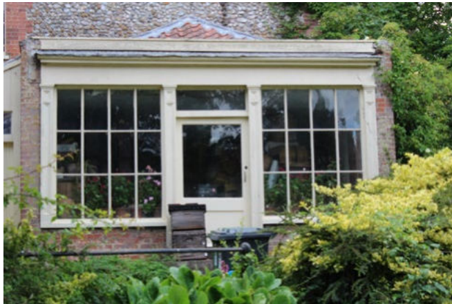
Nineteenth century shop unit located at Church House
