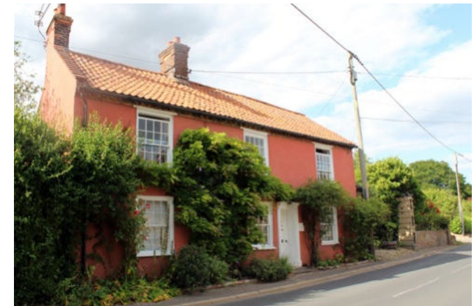
The Old Foundry House
