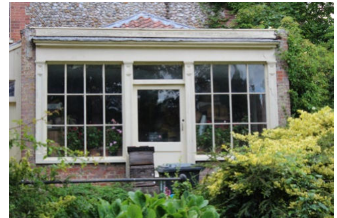
Converted nineteenth century shop front
