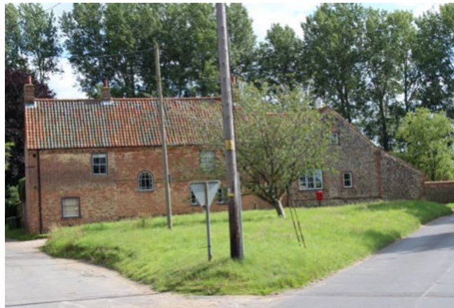
Dovecote and barn adjoin The White House Farm
