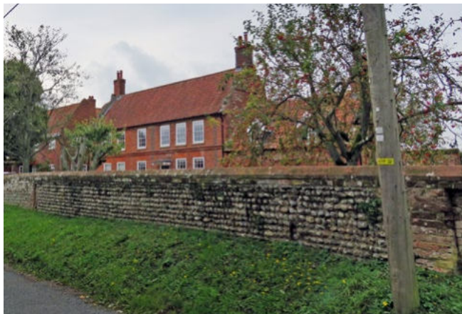
Historic cobble flint and brick wall
