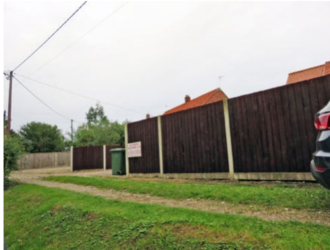
Timber board fencing
